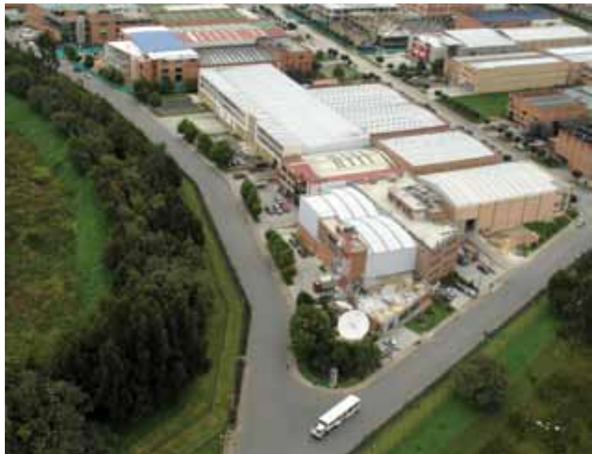
Zona Franca Bogota was officially inaugurated in March 1997 and now provides free trade zone services to a variety of companies and industry verticals.
